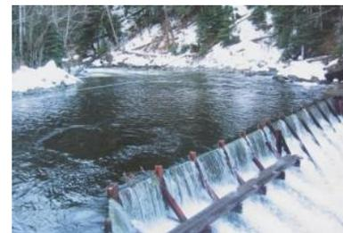
a capacity of 2 MW. In the winter, small run-of-river hydroelectric power stations don't run at capacity because most of the water is trapped in the snowpack. Run-of-river generating stations lack reservoirs behind their dams. While less disruptive to the environment, the power supply is not continuous when the flow of water is reduced.
